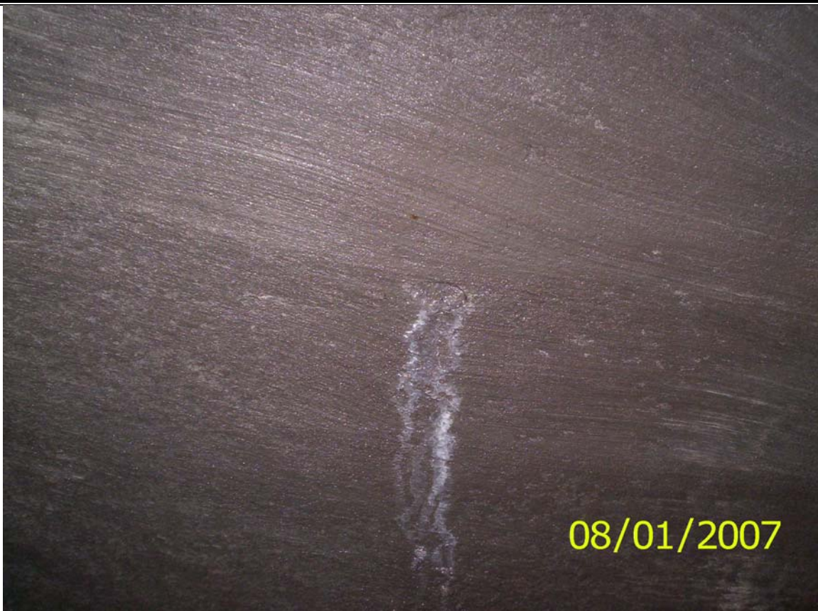
Brick Sewer Aftr Gunit Application
