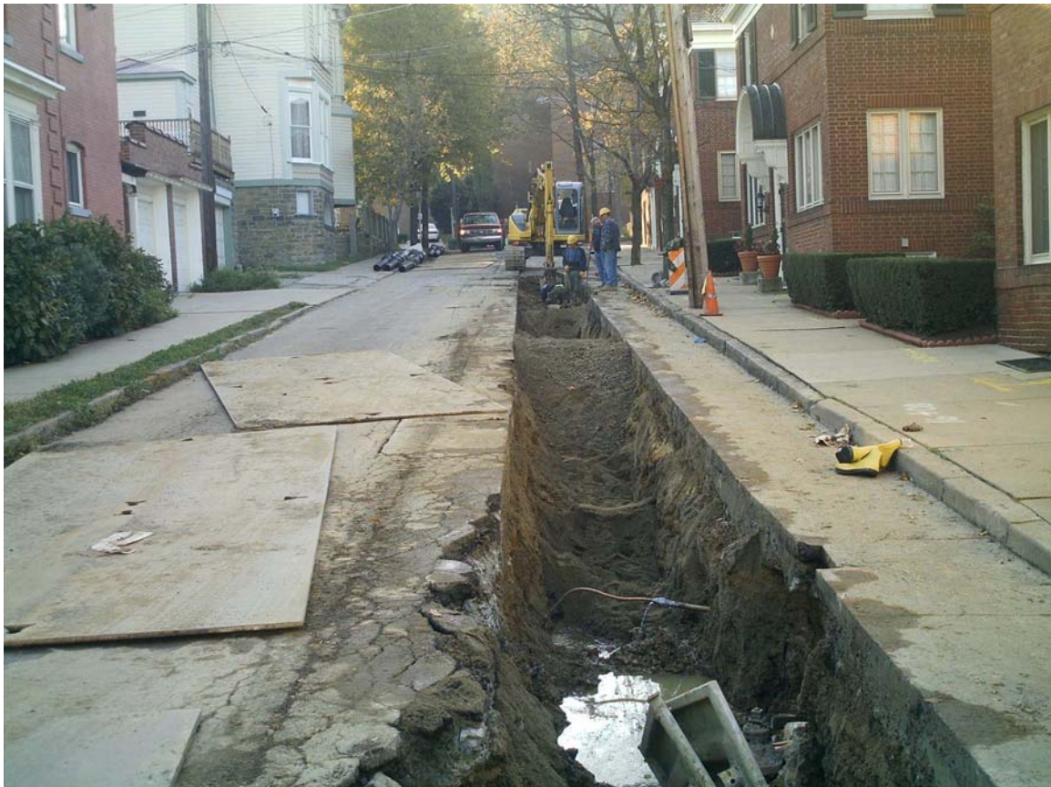
New Waterline Construction
