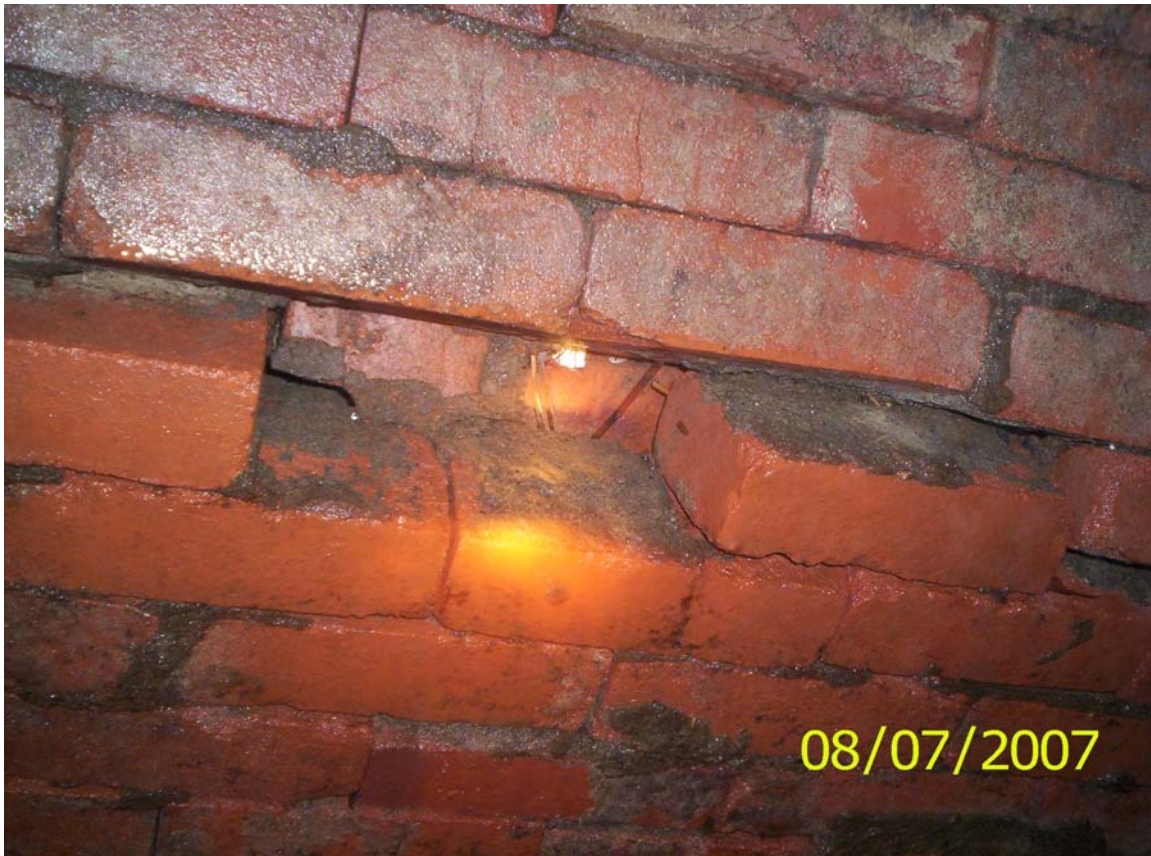
Existing Damaged Brick Sewer 1
