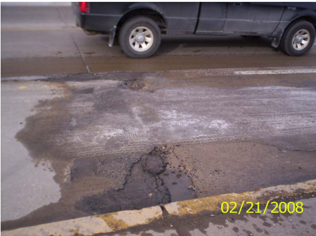
Icing on Roadway Due to Waterline Leak
