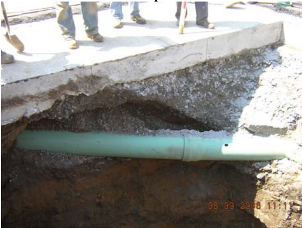
Completed Point Repair
