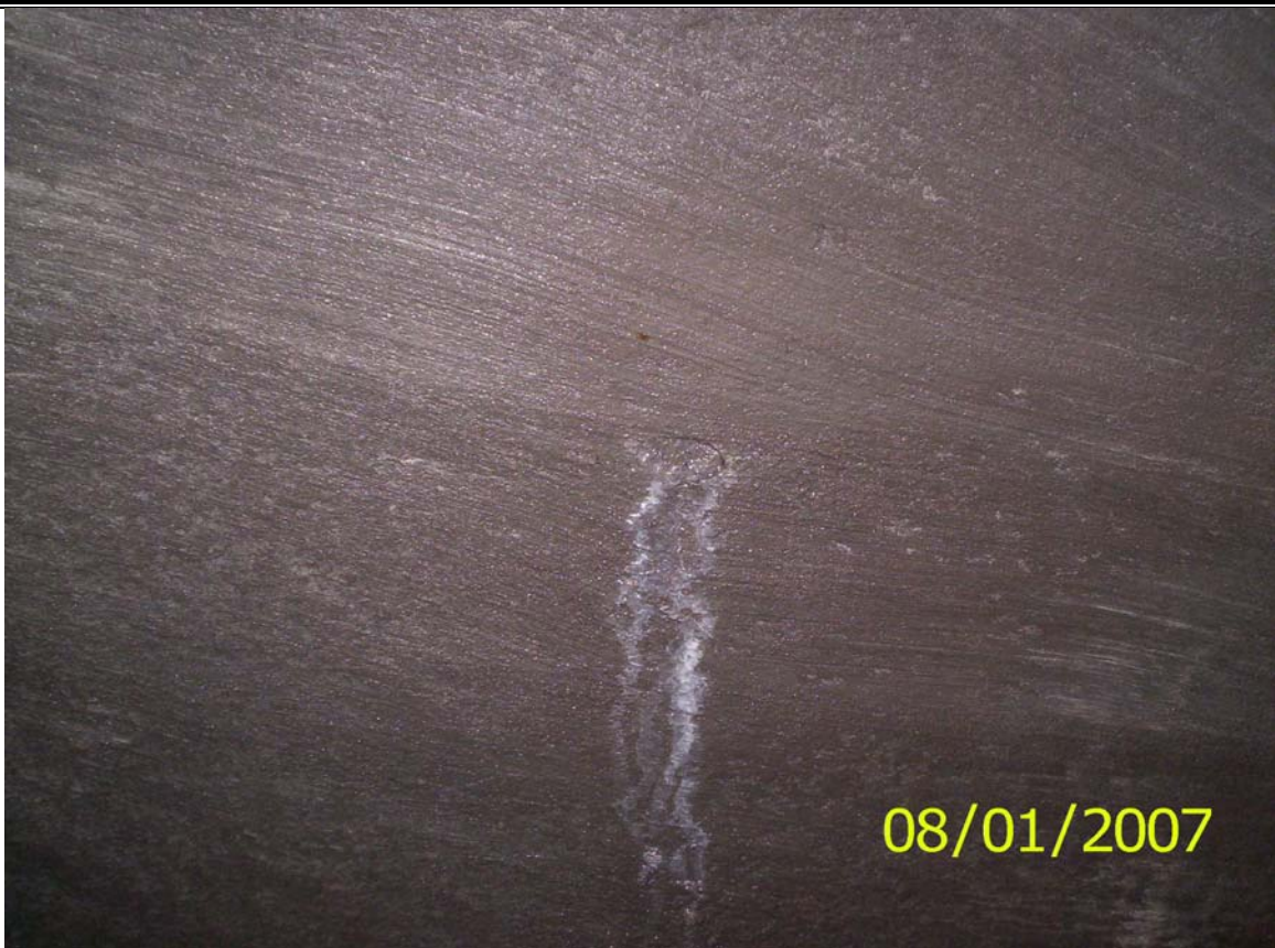
Brick Sewer Aftr Gunit Application
