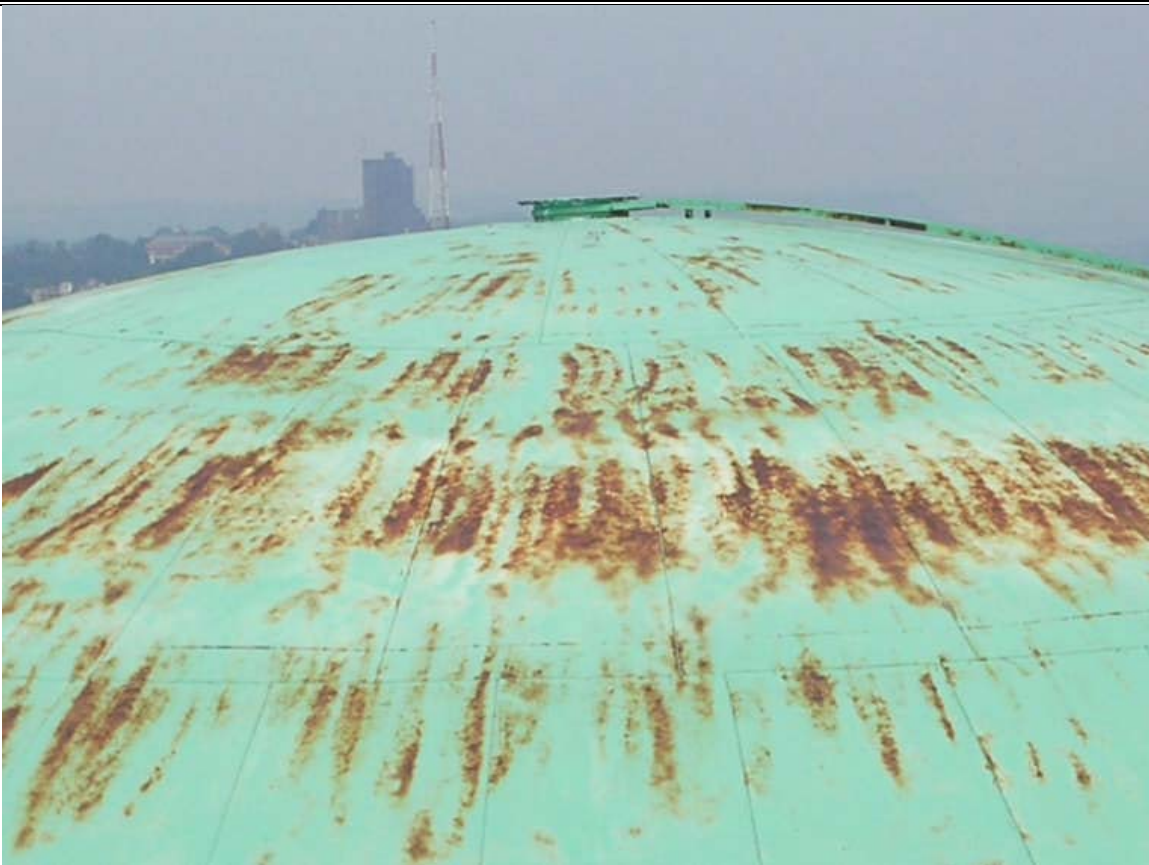
Corrosion of Allentown Tank Roof
