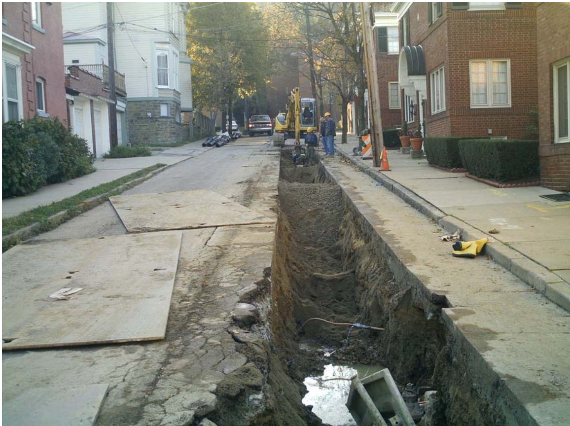
New Waterline Construction
