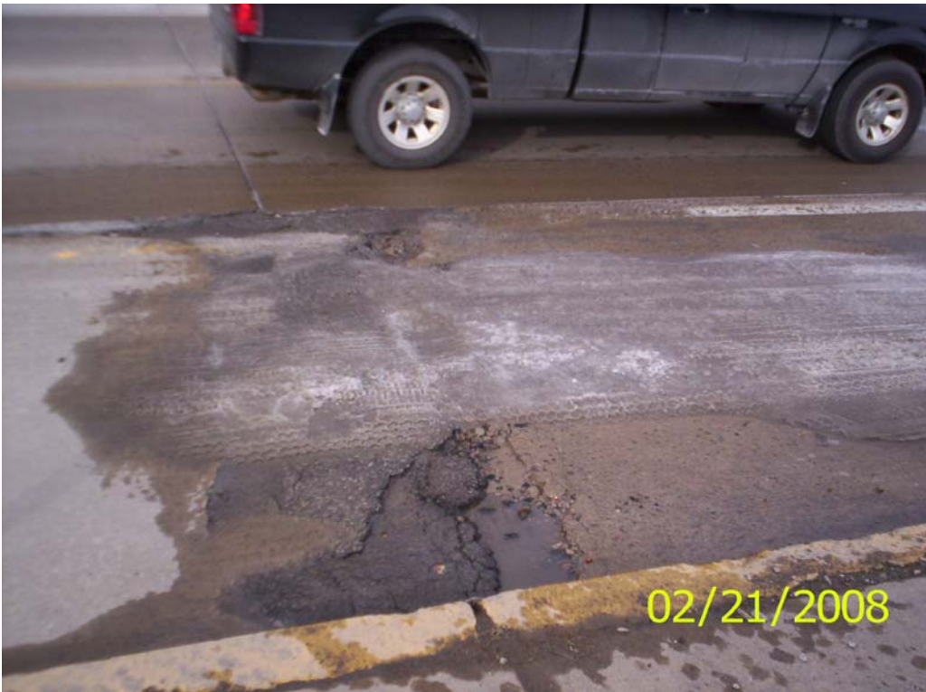
Icing on Roadway Due to Waterline Leak
