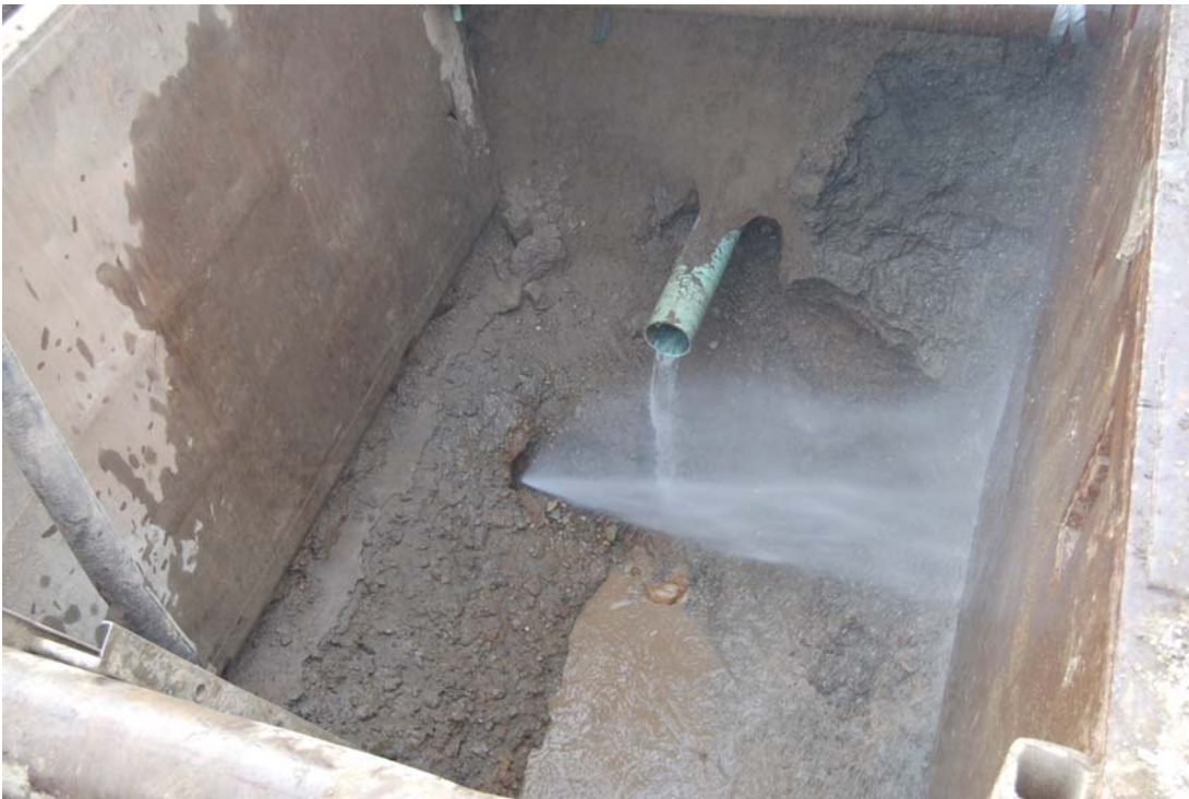
60-inch Water Main Leak
